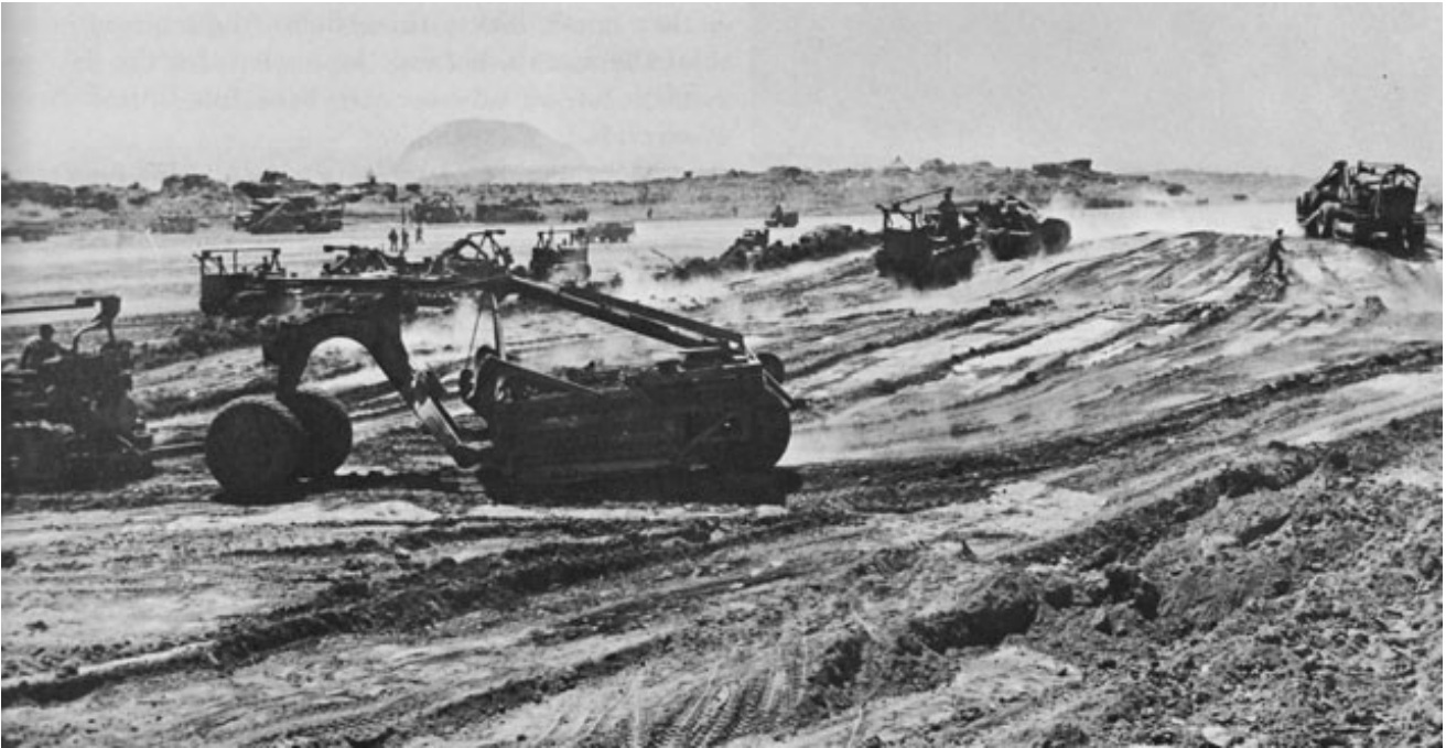
Construction of Tinian Airport
